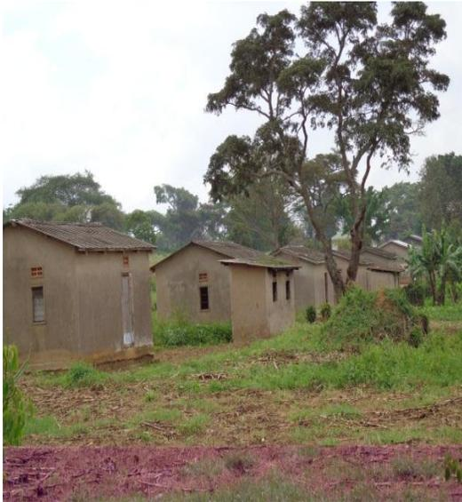
**Figure 6: Rwamwanja P/School staff quarters roofed with asbestos**
